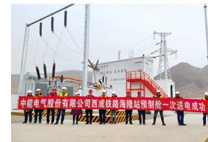
110kV Xicheng Railway Prefabricated Substation
