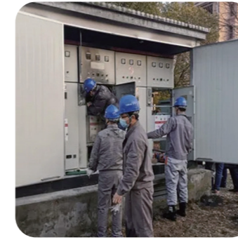
High maintenance cost
